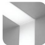
wall to ceiling corner
